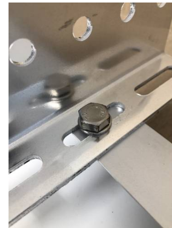
M8 module fixing
