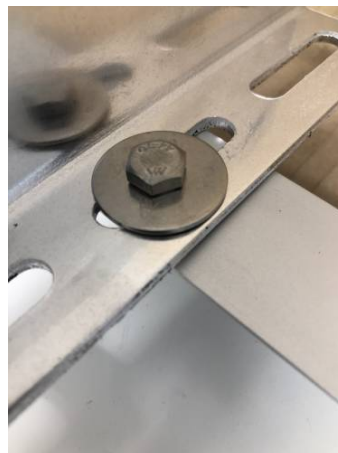
M6 Module fixing with penny washer
