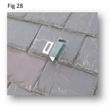
Using a standard roof hook on a slate roof
